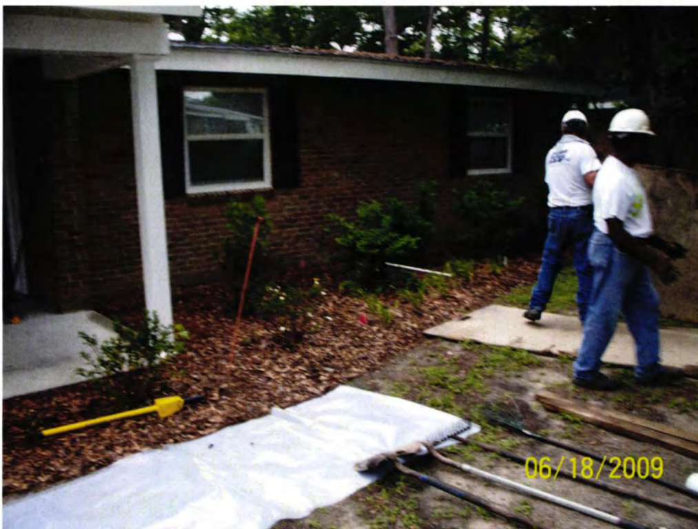
Picture 1: UST 1132Iris's location prior to excavation.
